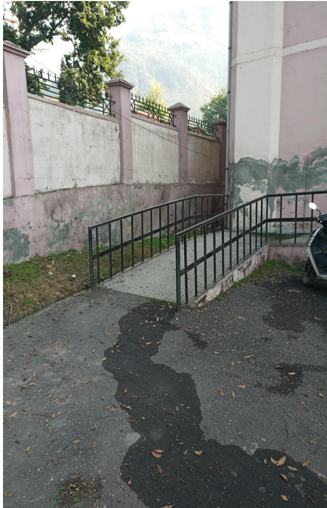
Ramp for Divyangjans
