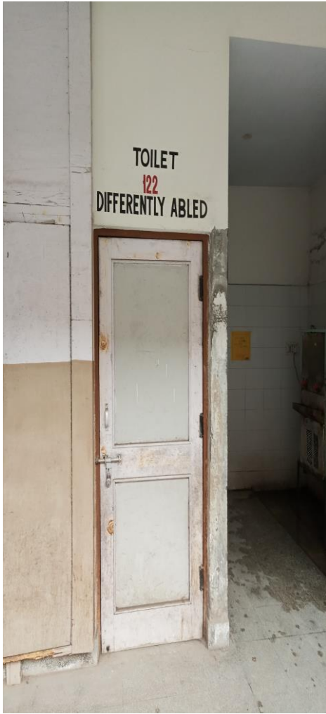
Toilet facilities for Divyangjans
